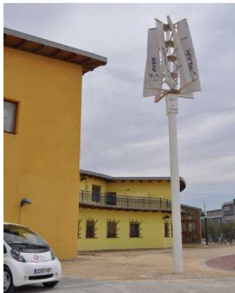
Fig. 5.8 Vertical axis wind turbine from Kliux energies ( http://www.kliux.com ), at CIRCE.
