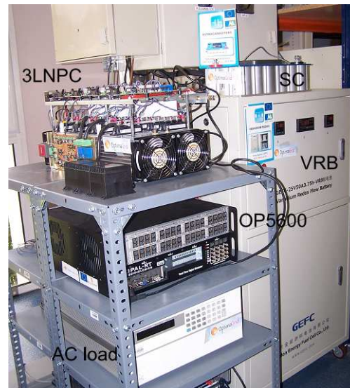
Fig. 3.6 Photograph of the experimental platform.
