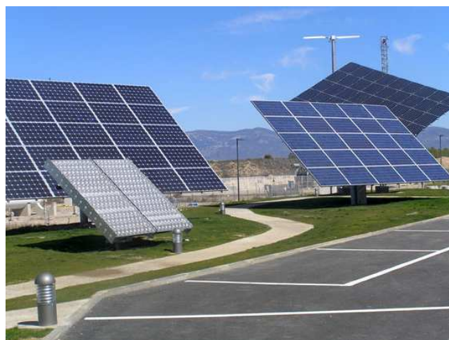
Fig. 1.4. DEGUER solar trackers and behind MECASOLAR solar tracker.
